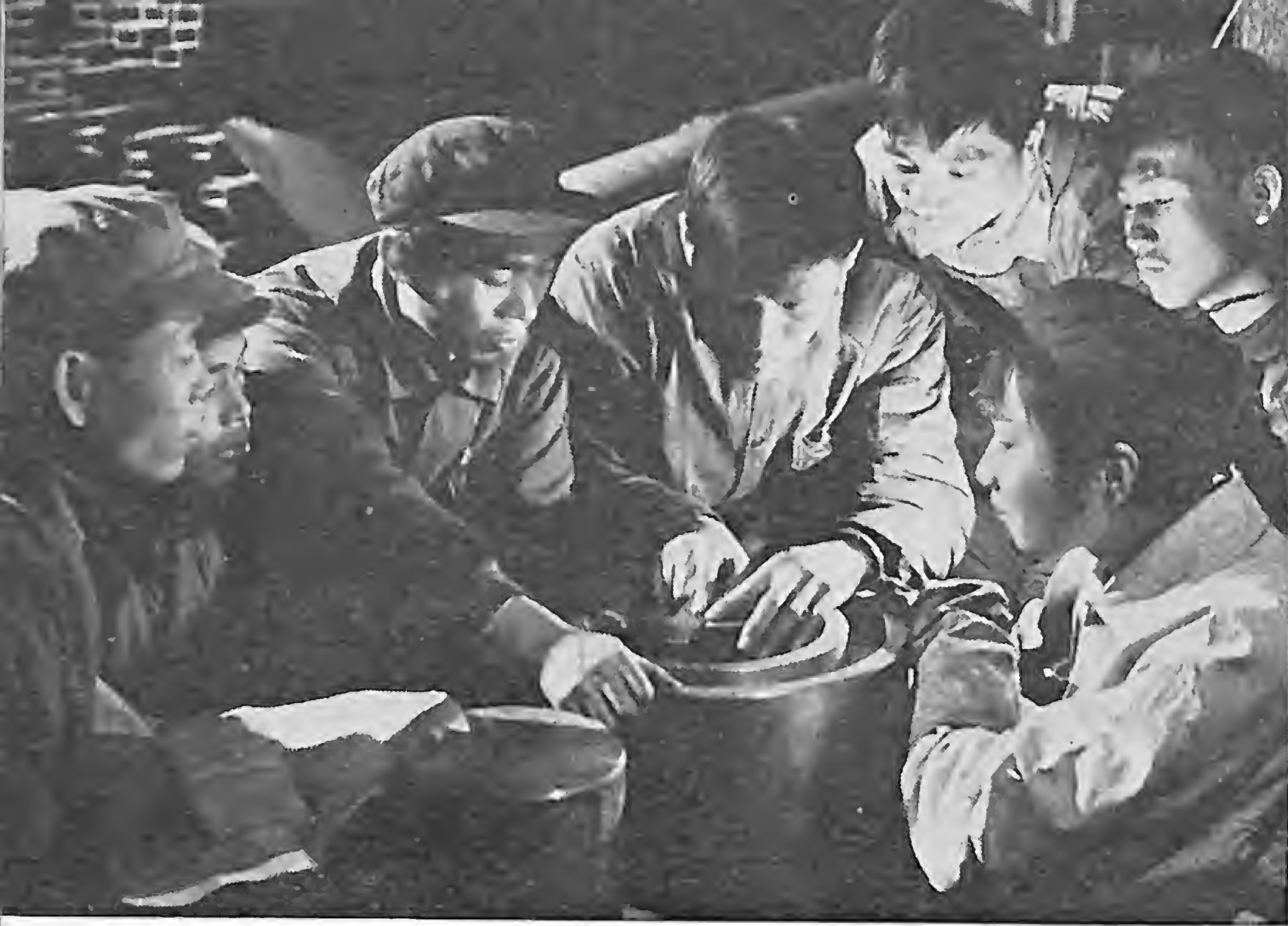
Workers discuss how to make the extrusion press.
